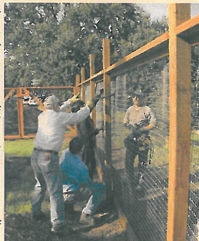
Tuesday Group workers install fencing around the nursery site
