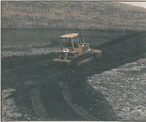
The bulldozer begins to deepen the pond
