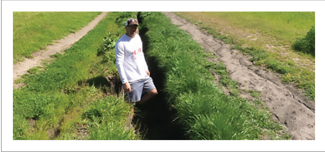
Storm damage in Shell Ridge —Mike Vickers, City Public Works Manager, stands thigh-deep in gully created by massive runoff from winter storms.
